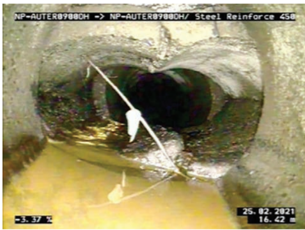
LEFT: A collapsed culvert pipe near the railway line at New Plymouth's East End.
